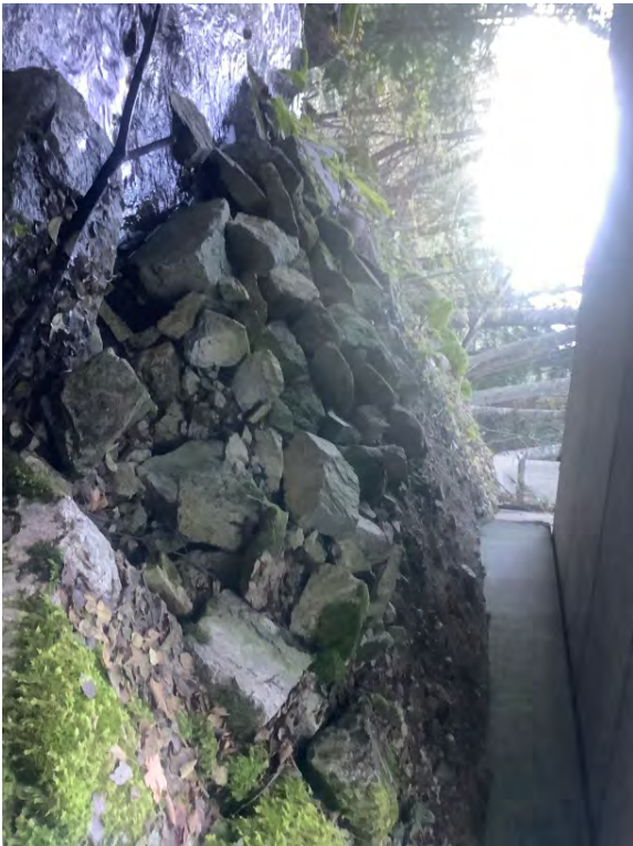
Right Bank Abutment when facing downstream
